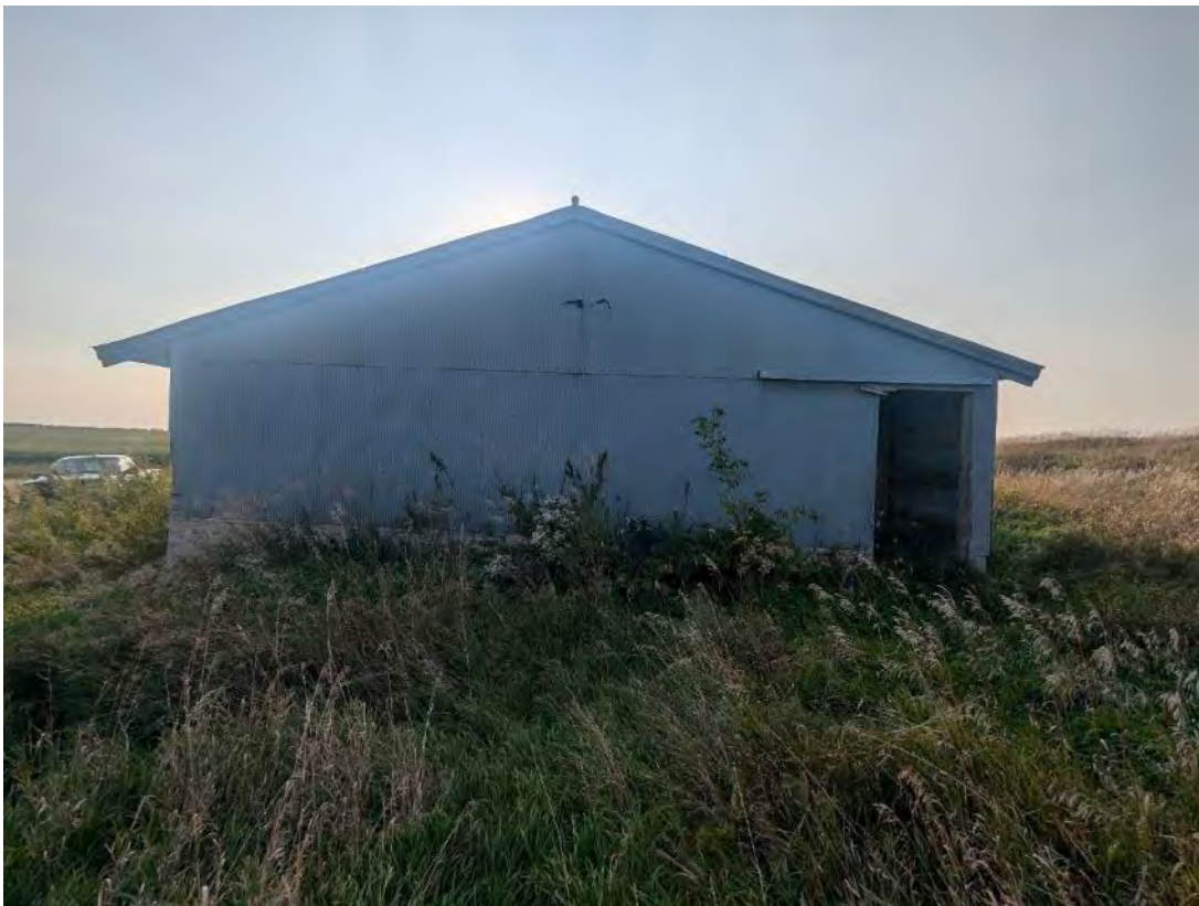
Figure 22. Farmstead 1 Standing Structure: West View.
