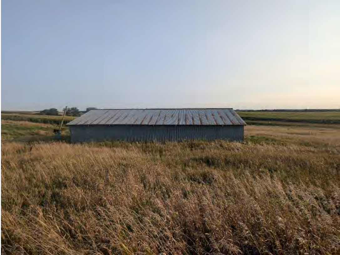
Figure 21. Farmstead 1 Standing Structure: South View.
